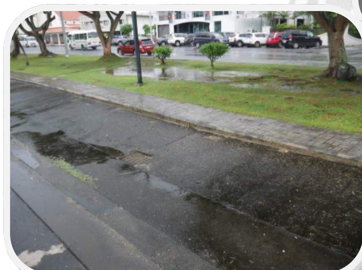
No. 7 Site—Beach Road at Old Court House.
